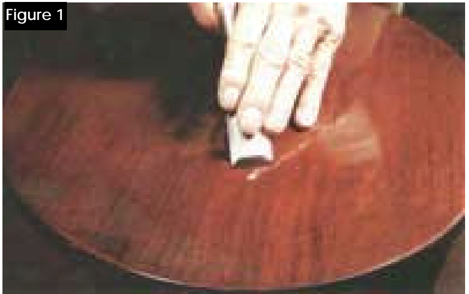
Figure 1: Use a very sharp chisel to shave away any “rim” around the edge of the defect, making the surface level.
